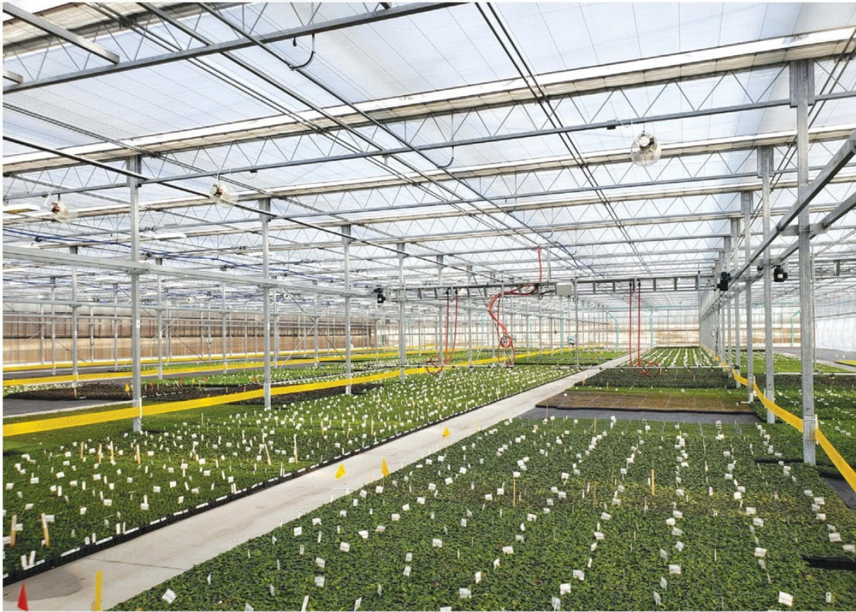
A retractable shade curtain that decreases but scatters sunlight can be especially useful when propagating plants.
